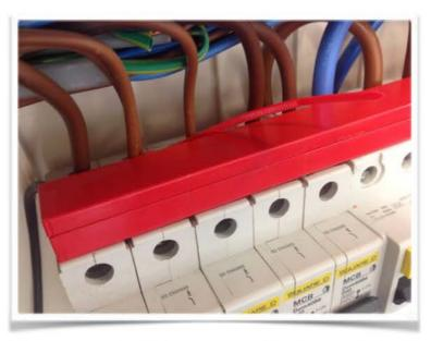
9. Once both cable ties are pulled tight the carriage should be secure and in close contact with the MCB connection terminals.
