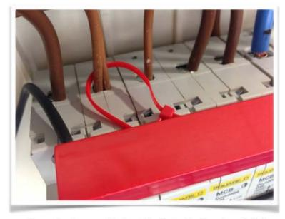
8. Once the free end is installed into the head, pull tight, ensuring that the carriage is held close to the outgoing circuit conductor.
