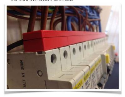
10. For the neutral bar place the supplied cable tie around the neutral bar. Please note that a separate T1150 device will be required for each neutral bar.
