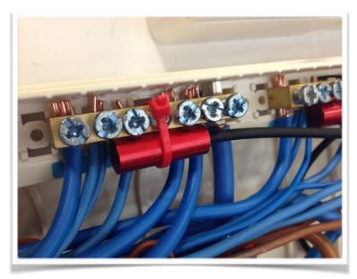
After fitting the Thermarestor system please ensure that <u>all</u> connections points within the consumer unit/distribution board are checked for tightness in accordance with manufacturers torque settings.
